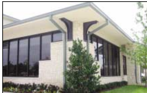
Fig. 5 Elegant corner of Dr. Adams's exterior finish synthesizes Austin limestone, glass, and steel.
